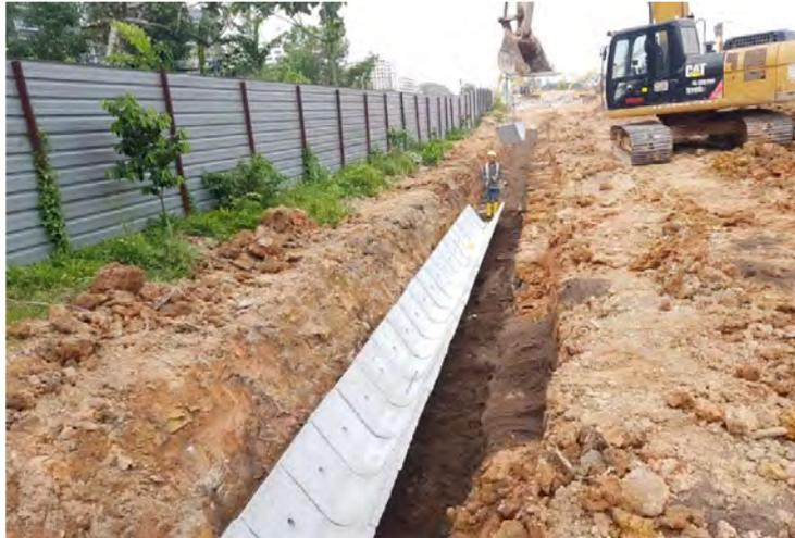
**Figure 7: Laying of C7 drain**
