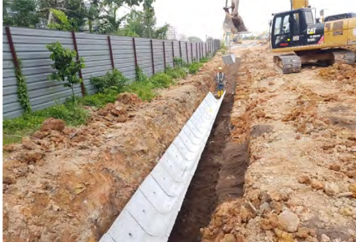
Figure 7: Laying of C7 drain
