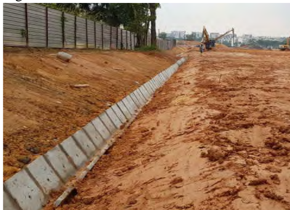
Figure 8: Compaction of slope adjacent to C7 drain
