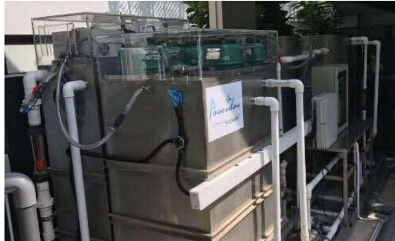
Above: Test-bedding of a decentralised blackwater recycling system for non-potable usage at JTC CleanTech One
