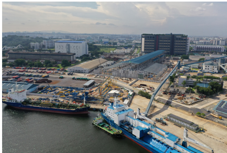
Below: Aerial view of the Ready-Mixed Concrete Ecosystem
