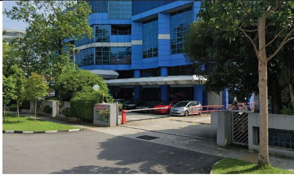
1 st Storey carpark next to main building with awnings/ canopies
