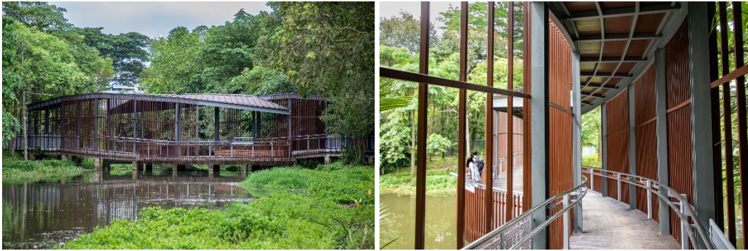
Photos credit: JTC
