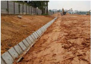
Figure 8: Compaction of slope adjacent to C7 drain
