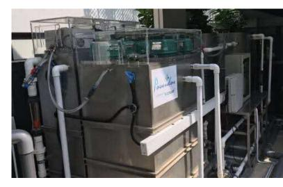
Above: Test-bedding of a decentralised blackwater recycling system for non-potable usage at JTC CleanTech One
